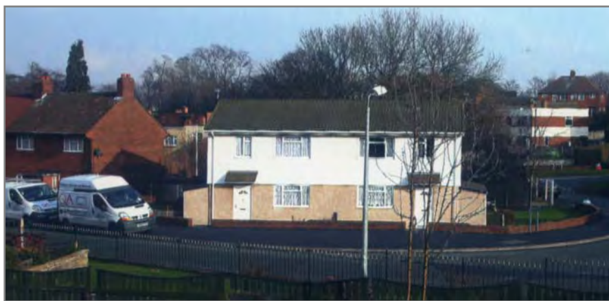
Arleston: three types of home. From the left: red brick 1930s Council houses; white painted 1948 'Airey' prefabs; flat-topped 1930s Air Ministry houses.
